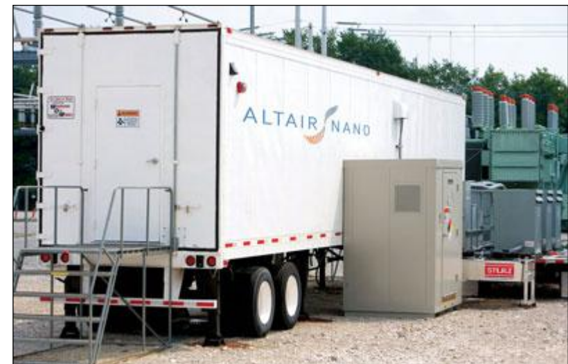
1MW Lithium Titanate Battery for A/S –PJM (Altairnano)
