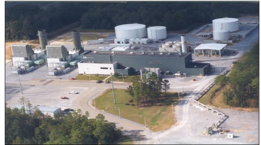
115 MW Compressed Air Energy Storage
