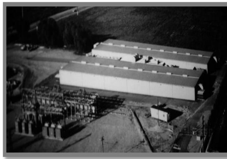
Energy Storage Peaker Substitution
